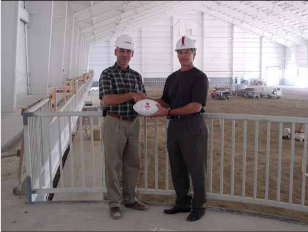
A game ball was presented each month to a member of the construction crew
